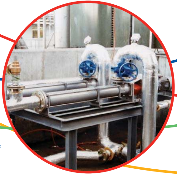
Pumping of slurry mix
